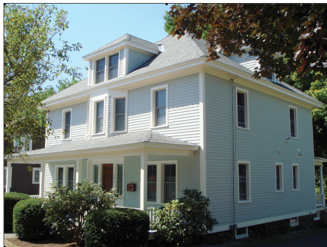
Photograph 1: 1912 Sears Craftsman House Retrofit— Super insulated retrofit done to an existing century old building in Concord, MA. Section shown in Figure 5 . This is what the future for existing buildings looks like.
